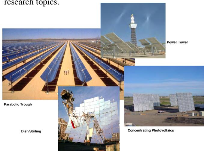
**Figure 17. Four different categories of concentrating solar power technologies: power tower, parabolic trough, dish/Stirling, and concentrating PV.**
