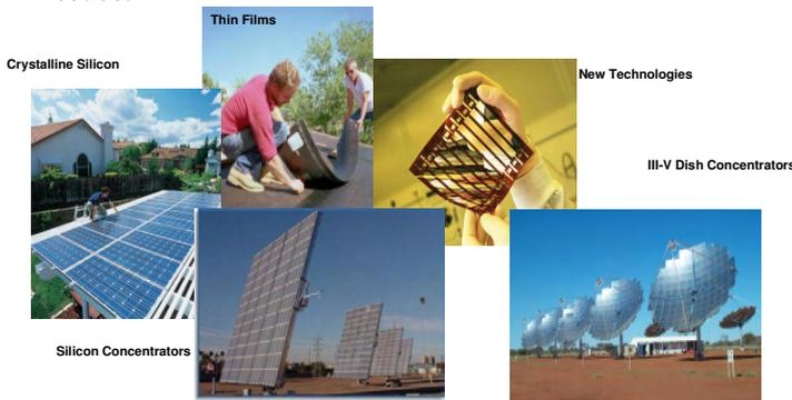
**Figure 14.** Various examples of photovoltaic technologies, from flat plates (crystalline silicon and thin-film devices, plus new second- and third-generation technologies) to concentrators (using silicon and III-V high-efficiency cells).
